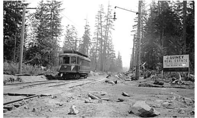
Figure 2.2. Vancouver's Fourth Avenue streetcar line freshly installed. Streetcars were provided before roads were improved or land subdivided for homes, as a necessary precondition for development. Here is the scene a few years before these other urban features were built. (Source: Michael Kluckner, Vancouver, The Way It Was . North Vancouver: Whitecap Books, 1984).
