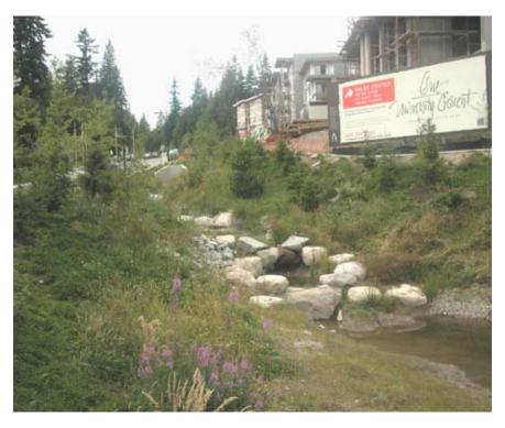
Natural drainage systems in which stormwater is held on the surface and allowed to seep naturally into the ground protects against downstream degradation such as streambank erosion and increased water temperature, which is a byproduct of conventional stormwater management systems. Using natural systems to collect and filter stormwater reduces infrastructure costs. This neighbourhood protects all streams and uses natural systems for stormwater management.
