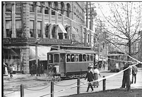
Figure 6-2: Historic photograph of a streetcar in Vancouver, ca.1900. 3
