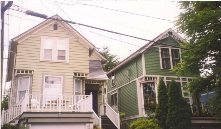
Two small lot single family homes, Southeast Portland
